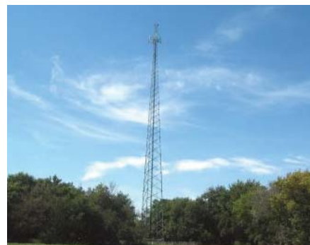
Figure 1. This is a photo of a new type of RF telemetry system that is now being marketed. This type of system establishes numerous miniature communication cells where the individual remote units communicate to and from the central recorder via predetermined cells. The individual remote units connect with their individual cell via spread spectrum communications. Each individual cell is then linked to the central recorder for command and control of the spread.
