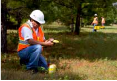
Lightweight, cable-free nodes are quickly, safely deployed, and their position is recorded for quick and easy retrieval.
